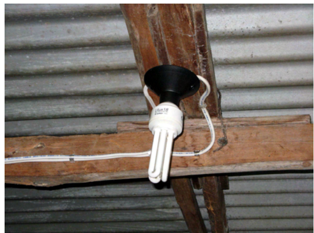
Solar lamps were installed in each room
