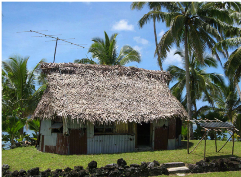
Radio hut with VHF antenna and solar panel in the foreground
