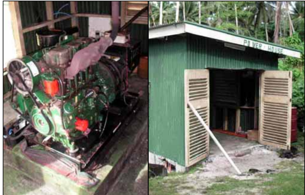
Figure 9: Generator and Powerhouse on Rotuma
