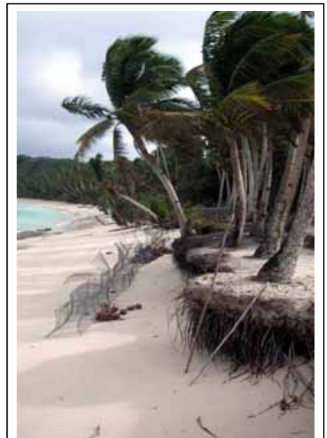
Figure 3: Costal erosion near Motusa
