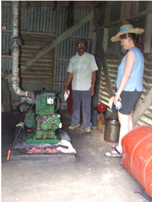
(a) Diesel generator in Juju.
