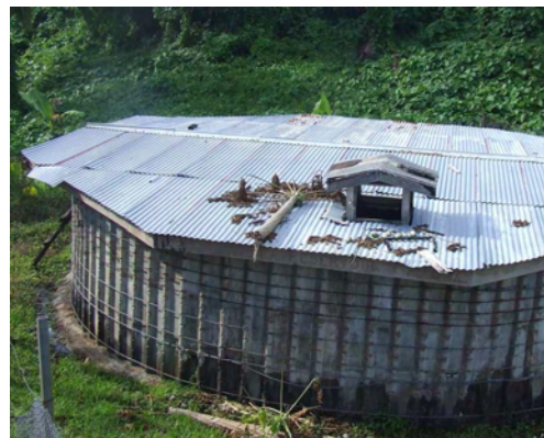
(b) Water supply reservoir. The tank holds 180m 3 .
