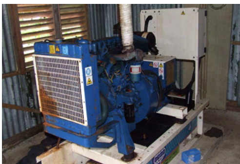
(a) FG Wilson Generator set.
