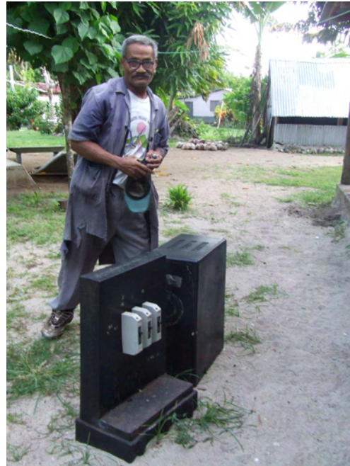
(b) Electricity grid substation in Juju.
